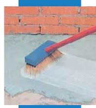
Applying cement slurry modified with Planicrete SP
