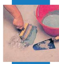
Floor patching: application of slurry
