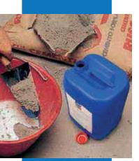
Mixing cement mortar with Planicrete SP for tile fixing
