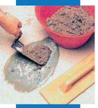
Floor patching: application of mortar
