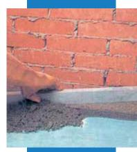
Applying cement screed modified with Planicrete SP
